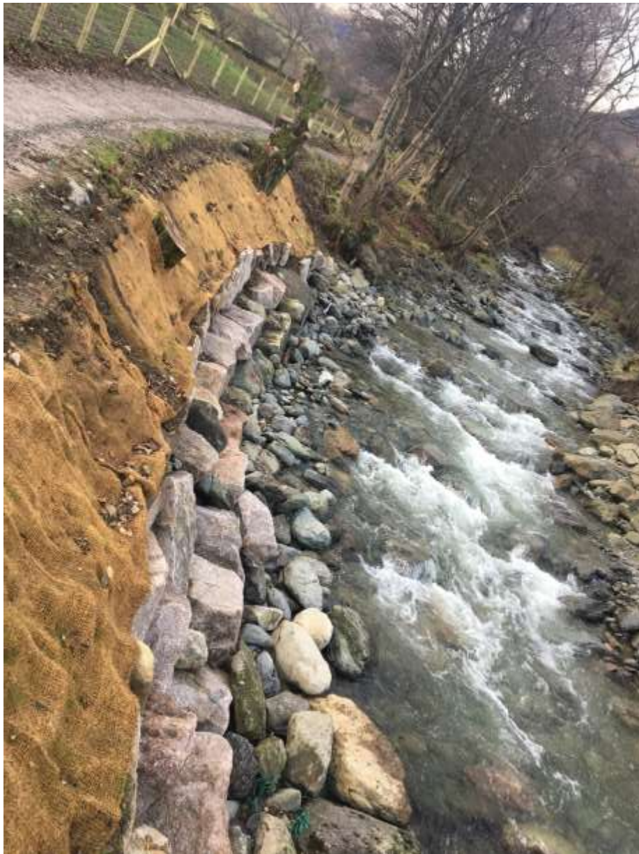
Freshly completed CFG/LDNP work on Gillside Footpath
