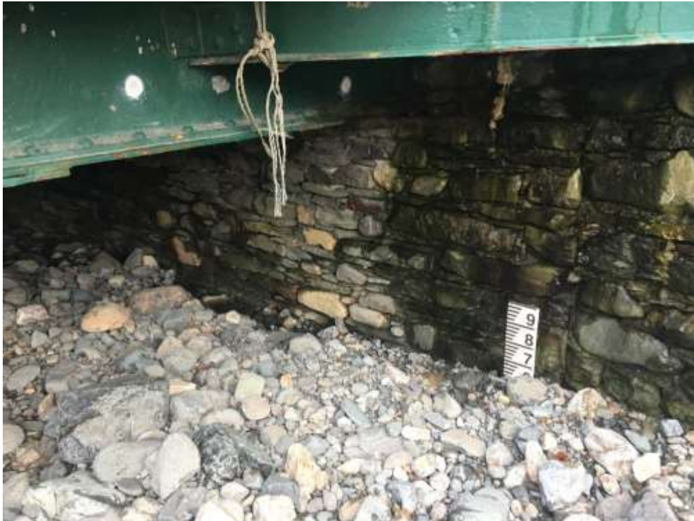
Glenridding Bridge Depth Marker – “Right Hand Side” looking downstream
